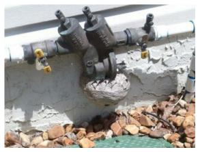
As I walked around the house to test the backflow device shown above..Booyah! There is a Hornet's nest on the relief valve. Did the relief valve open above 2.0? Yes, three months later.
