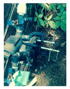
In the above picture someone put a different thicker gasket in place of the original Febco diaphragm and I'm guessing after tightening the bolts with the thick gasket it still leaked so.. What's a man to do? Break out the good ole C-Clamps and not 1 but 3!
